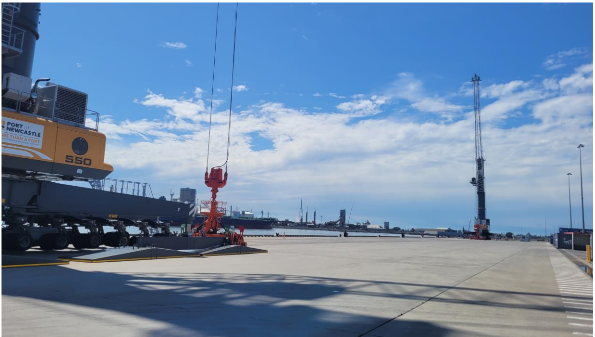
Photo 2: Mayfield 4 Berth facing south east
