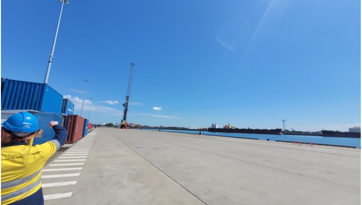
Photo 1: Mayfield 4 Berth facing north west
